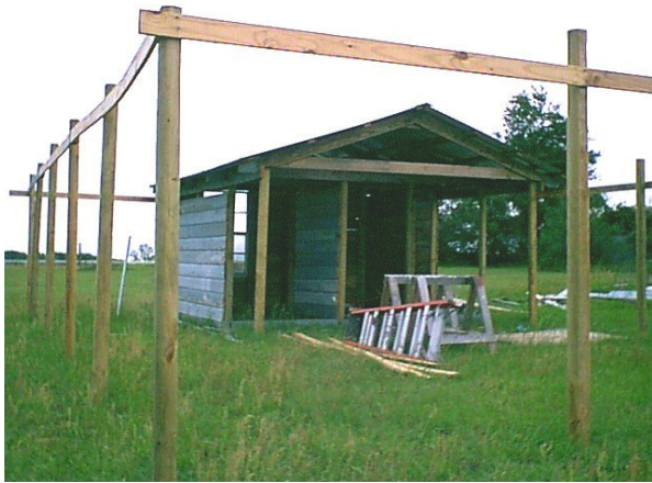
Building the chicken house and yard back then.
