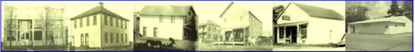
The Waller Masonic Lodge Buildings From December 30, 1897 To The Present
